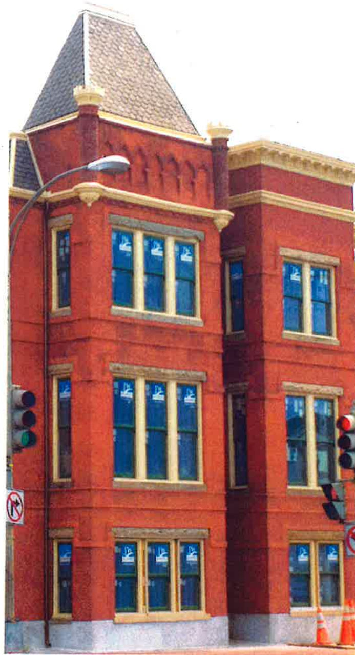
Rhode Island Avenue at New Jersey Avenue, NW
